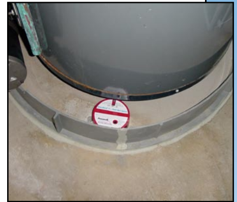
FloodRing™ around a water heater, showing optional WaterWatch® Alarm.
